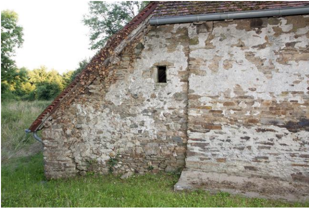
Figure 9 : Issue secondaire (façade nord)
