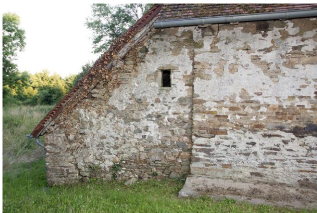
Figure 9 : Issue secondaire (façade nord)
