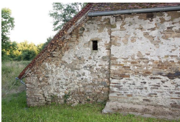
Figure 13 : Issue secondaire (façade nord)
