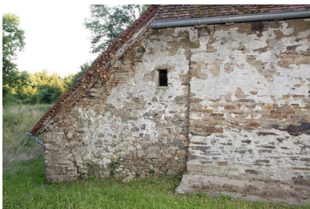
Figure 13 : Issue secondaire (façade nord)
