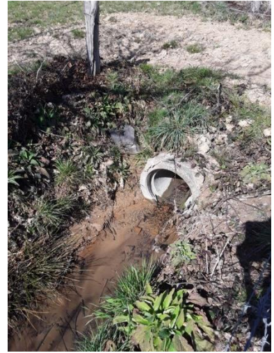
12 – Buse Ø500 passage agricole
