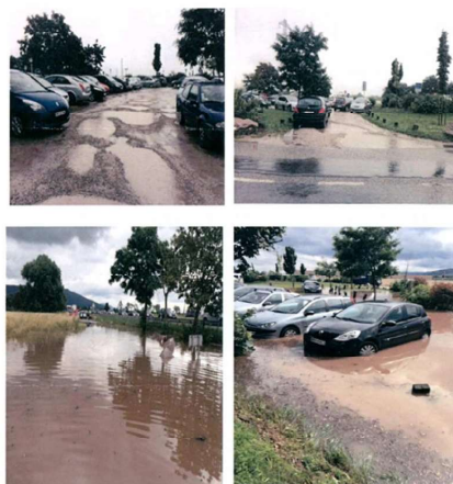
Figure 1-2 : Inondations au parking Grube
