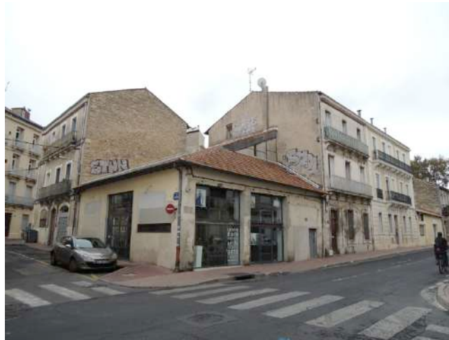
Restructuration de hangar
