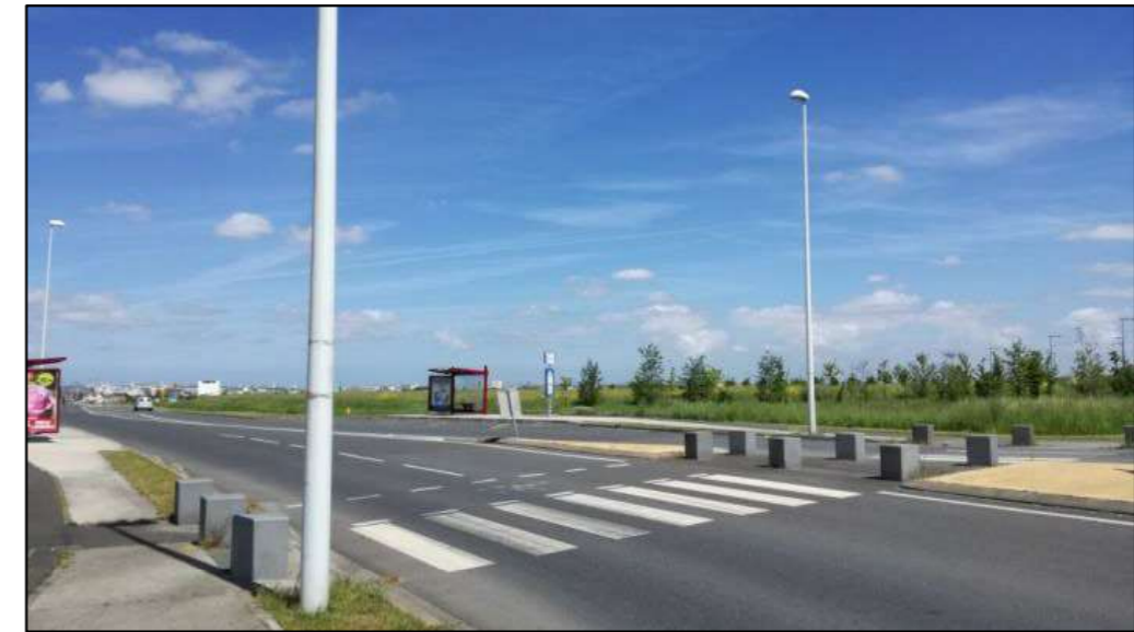
Figure 154 : Route RD 562A
