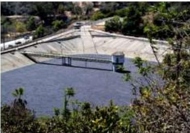
Installation is incredibly quick and easy. When settled into the water the additional stability is able to cope with wind speeds in excess of 147km/h (48m/s) preventing balls being blown from the surface.
