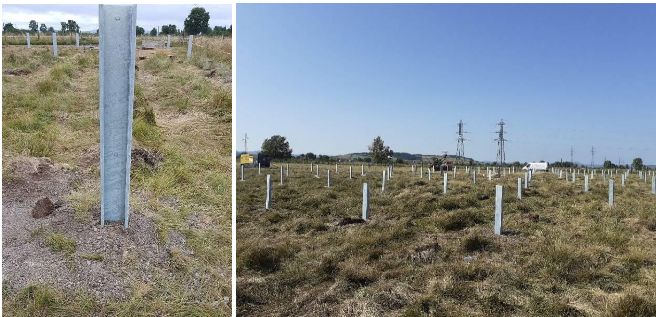
Photo 3 : Exemple de pieux forés (BORALEX)
